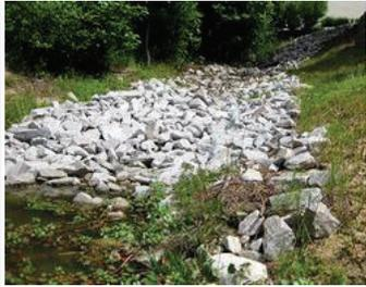
of the basin's embankment where water can leave the pond during an extreme storm or rain event. These areas can be stabilized with concrete, rip-rap or herbaceous vegetation. The emergency spillway should be kept clear of trees, sediment, and debris. They need to be checked for any erosion or structural weaknesses.
