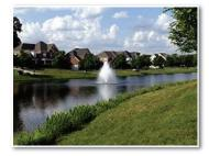
sediment and pollutants, and then release the water slowly to mimic run-off from the site before development. These ponds not only function as stormwater management facilities, but are often designed as key features in communities. Most of these ponds have similar basic parts:
