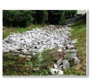
of the basin's embankment where water can leave the pond during an extreme storm or rain event. These areas can be stabilized with concrete, rip-rap or herbaceous vegetation. The emergency spillway should be kept clear of trees, sediment, and debris. They need to be checked for any erosion or structural weaknesses.
